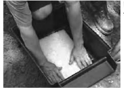
Lay the filter mats in the bottom of the filter box on top of the support tubes or support stands depending on model.
