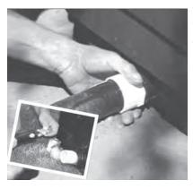
Glue the PVC flex pipe into the male adapter and hold together until glue is set.
