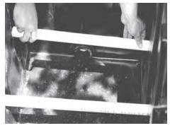
Insert the PVC support tubes into the "V" shaped notches in the bottom of the filter on the Prelude and Melody models, the Sonata and Symphony models have built in supports instead of the PVC pipe. Be sure filter does not move while backfilling with dirt around it.
