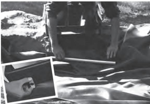
Run the protective underlayment in the pond and up the stream (if one is installed). The underlayment should overhang the stream bed and be up to the bottom of the filter box. Lay the liner in the pond over the underlayment. Work as many wrinkles out of the liner as possible. The liner should be run up the stream or to the filter box.
