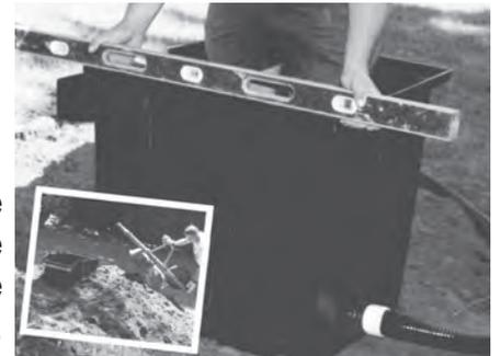
Set the filter box on the prepared surface. Be sure filter sits level side to side and tips forward 1/2" to 1".
