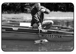
9. Use rope looped around diffuser to assist lowering assembly to pond bottom.
