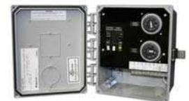
Each unit includes a UL Approved, 240V Power Control Panel complete with Class A Human Rated GFCB, 24 Hour Mechanical Timer, Surge Protector, and 24 Hour Timer for the optional lights. NEMA Type 3r/4x Thermoplastic enclosure.
